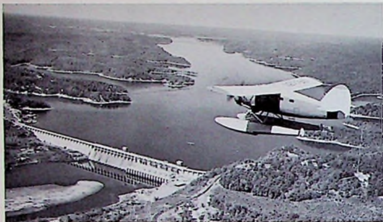
AIR VIEW OF BAGNELL DAM WHICH CREATES LAKE OF THE OZARKS.
